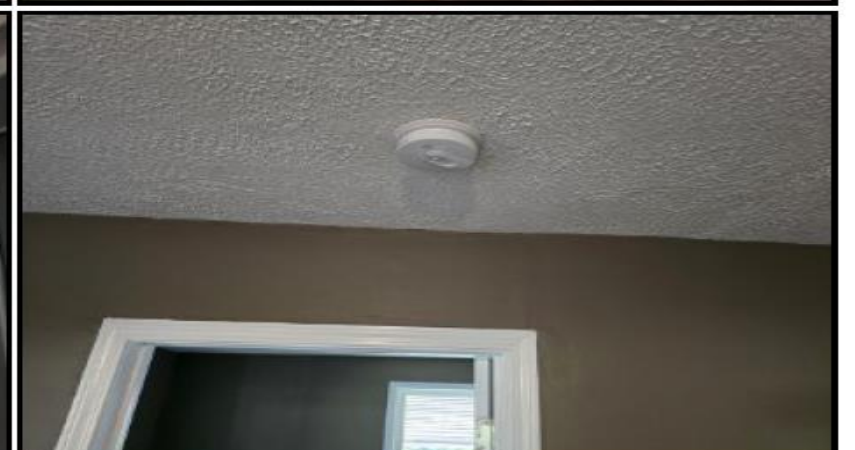
Smoke detectors installed at proper locations.
